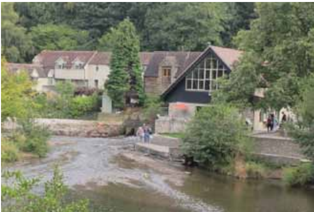
Stone revetments beside the Green Café on the former site of Castle Mill © Michael Rosenbaum
