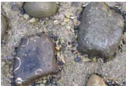
Cobbles set in cement © Michael Rosenbaum
